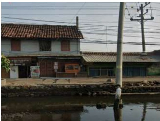
Figure 4. Condition of Elevated and Non-Elevated Houses. Source: Researcher documentation
