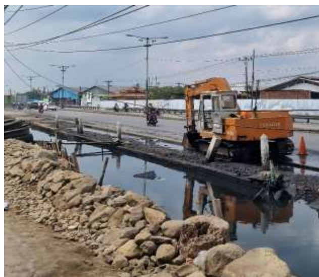
Figure 10. Dredging Sedimentation Source : Researcher Documentation , 2025
