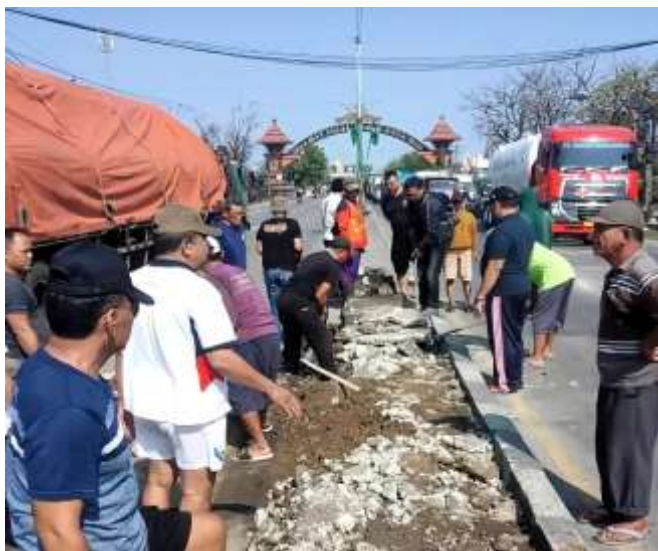
Figure 7. Road demolition carried out by residents. Source: Researcher documentation.
